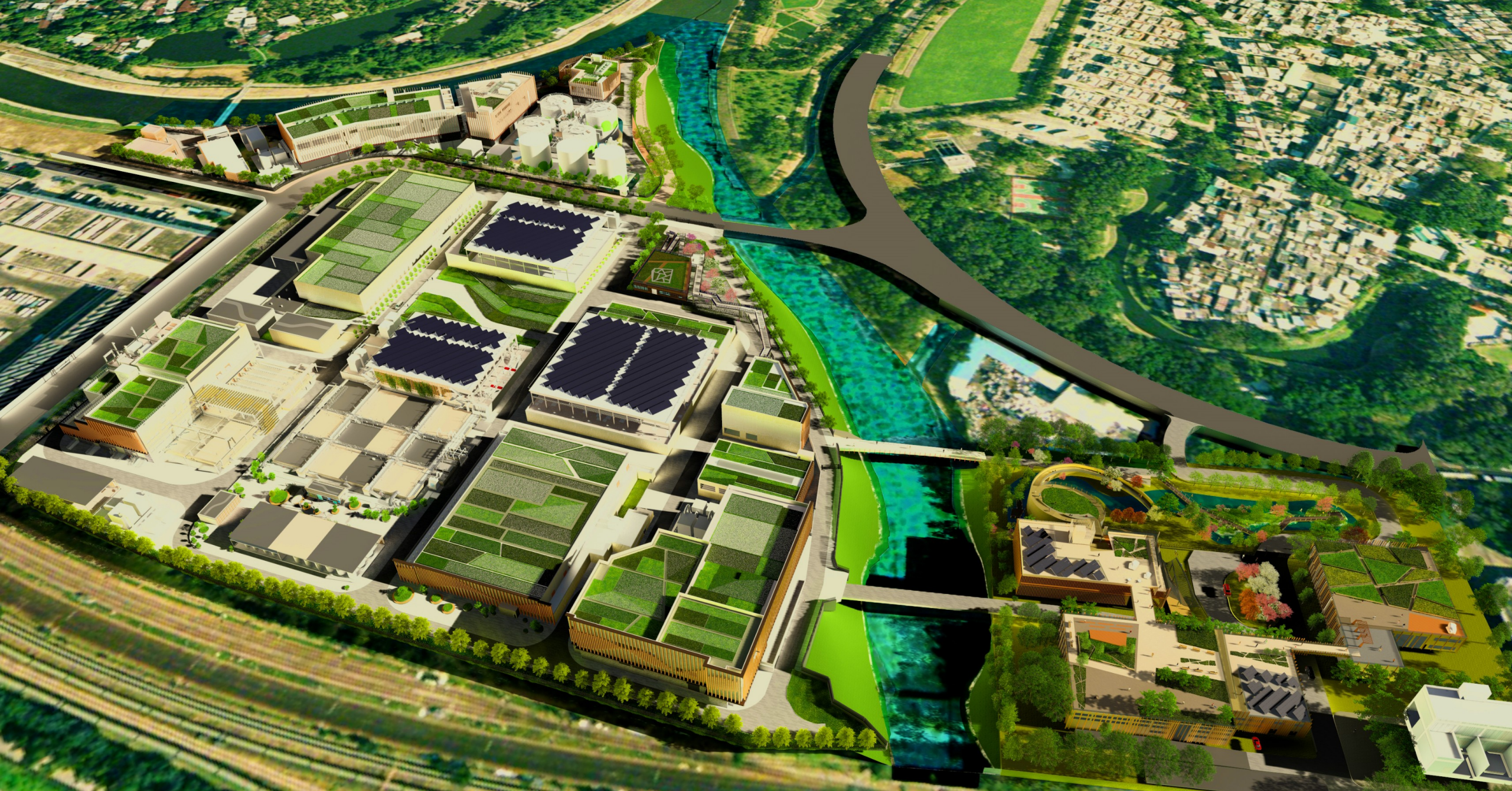
Shek Wu Hui Effluent Polishing Plant, Hong Kong
