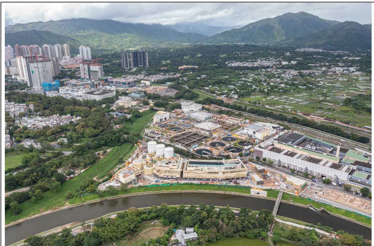
Description: Aerial Photo in Portion C on 16 July 2024
