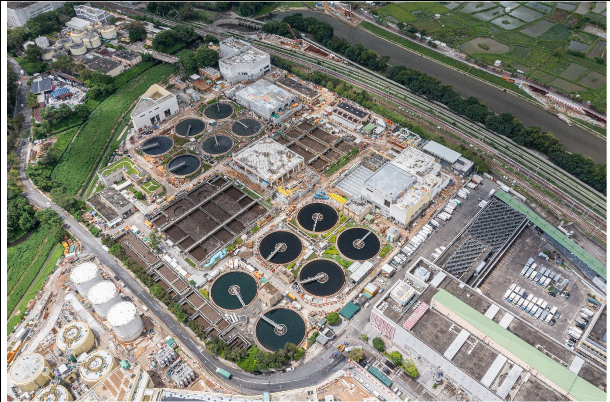
Description: Aerial Photo in Portion A & Portion B on 16 July 2024
