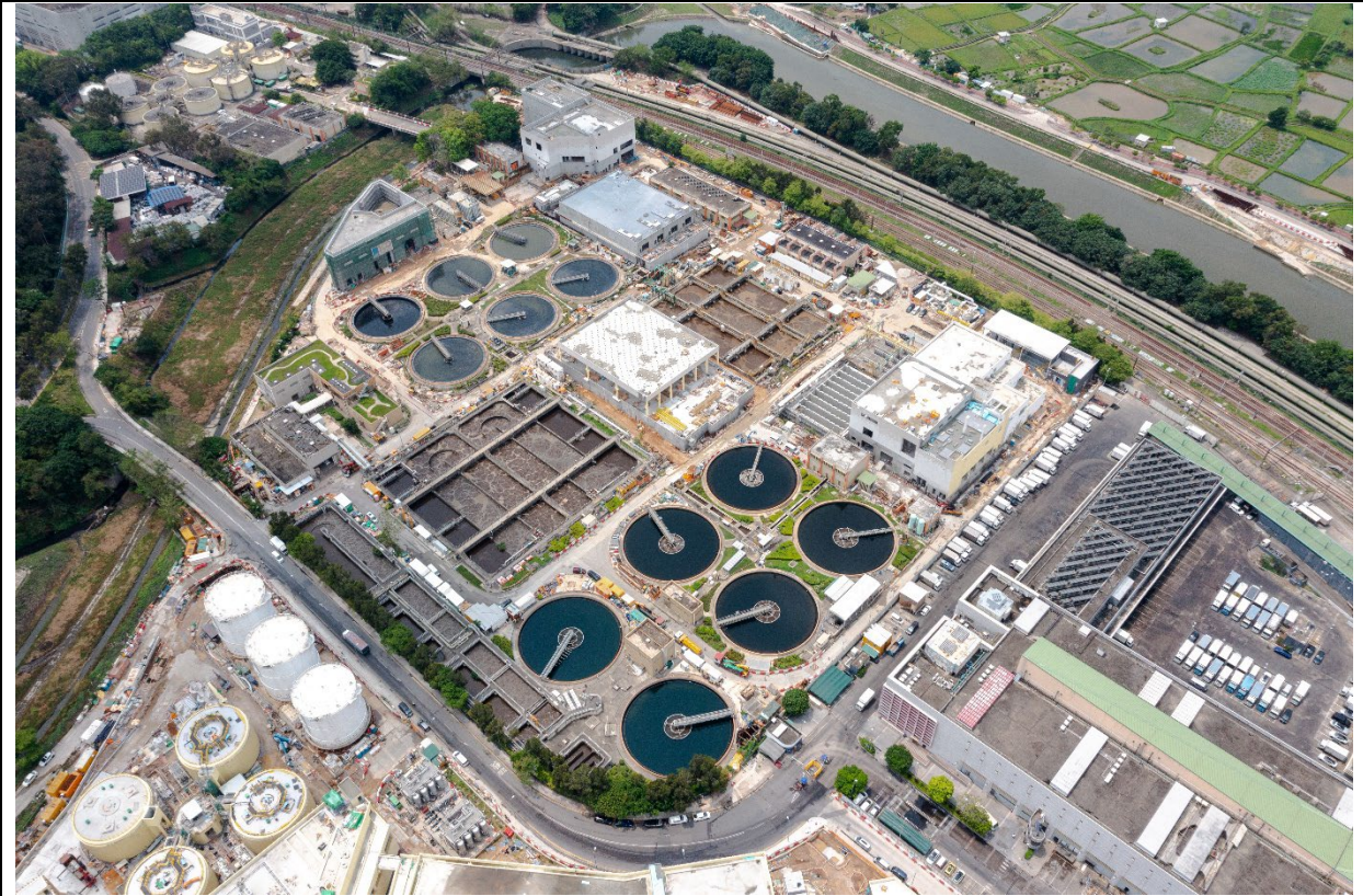
Description: Aerial Photo in Portion A & Portion B on 19 April 2024
