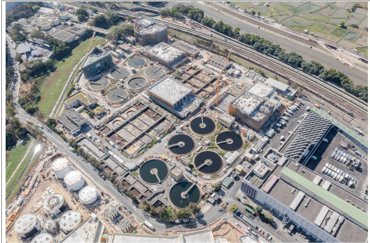
Description: Aerial Photo in Portion A & Portion B on 22 January 2024
