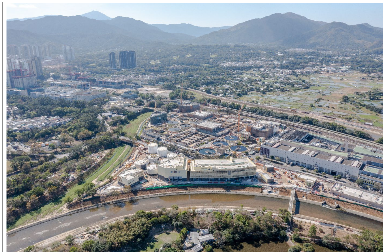
Description: Aerial Photo in Portion C on 22 January 2024
