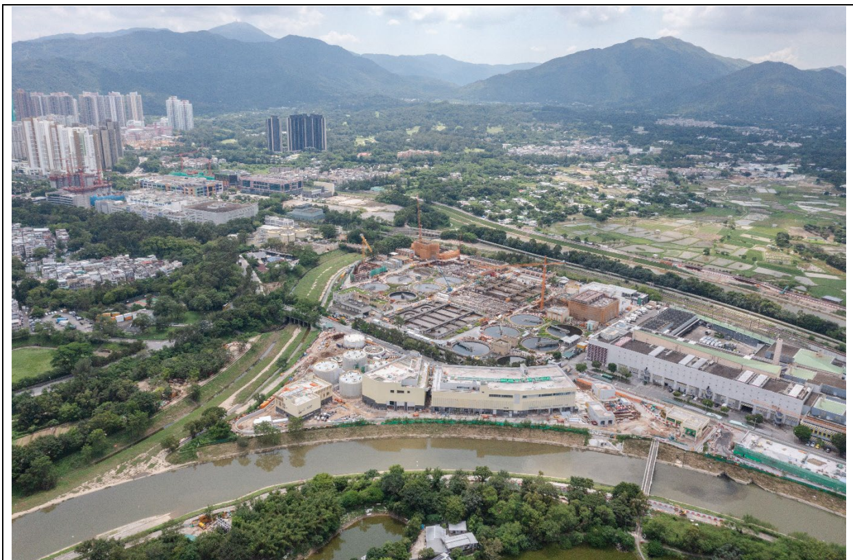
Description: Aerial Photo No. 2 in Portion C on 23 September 2023
