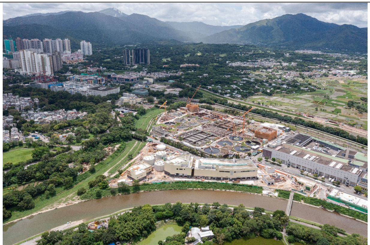
Description: Aerial Photo No. 2 in Portions C on 21 August 2023
