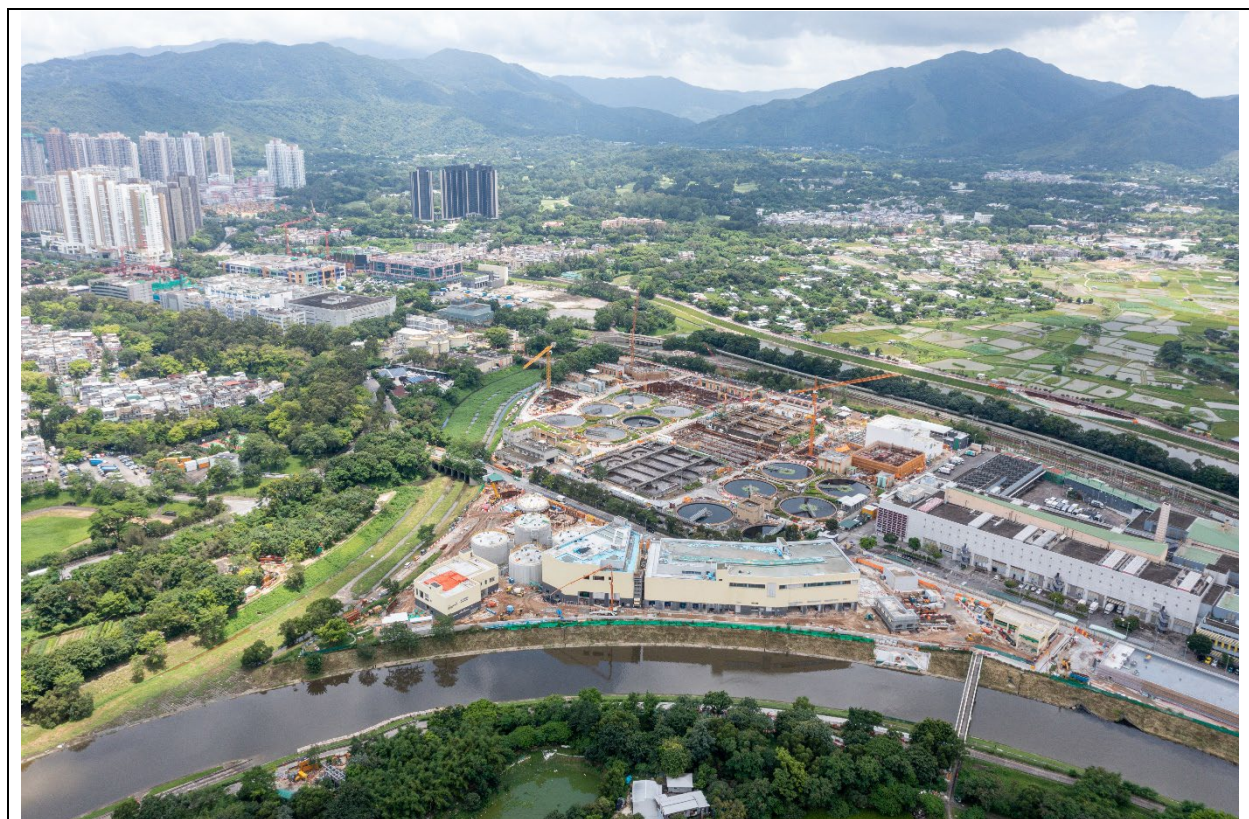
Description: Aerial Photo No. 2 in Portions C on 20 June 2023
