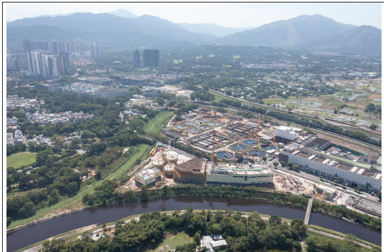
Description: Aerial Photo No. 2 in Portions C on 21 October 2022
