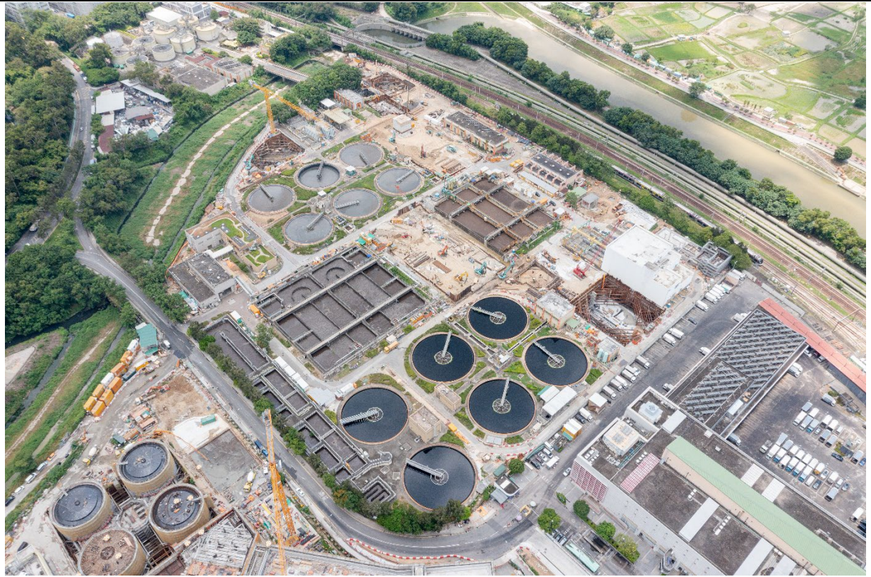
Description: Aerial Photo No. 1 in Portion A & Portion B on 26 July 2022
