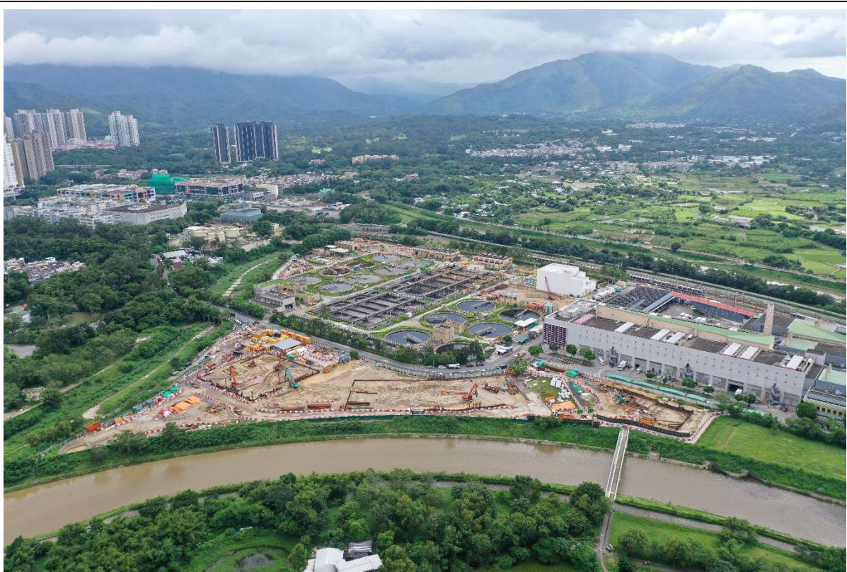
Description: Aerial Photo No. 2 in Portions B & C on 21 Sep 2020
